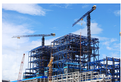
Steel Construction / Civil Engineering
