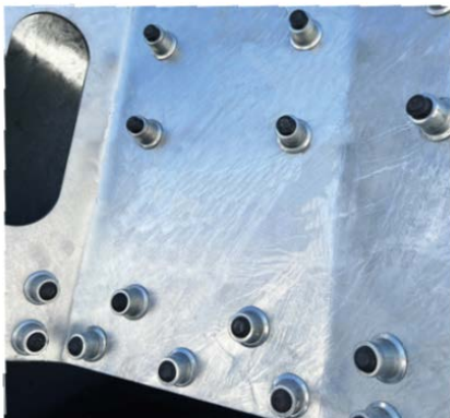
Installed C50L Huck Fasteners in Screening Equipment
